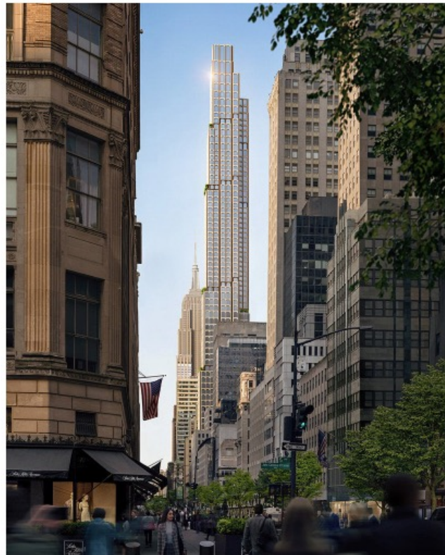
Fifth Avenue's tallest residential tower is backdropped by the Empire State Building
