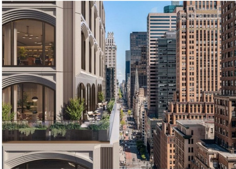
residences open onto gardened outdoor space as tiered terraces spiral up the tower
